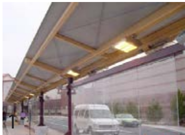
BRT heated shelter
